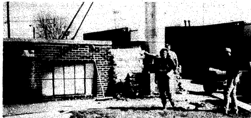
Volunteers Kathy Skinner, Randy Lanning and A.J. Johnson work on the windows and walls of the former Wakefield High School which now houses the Humpty Dumpty Day Care and the Senior Center.
